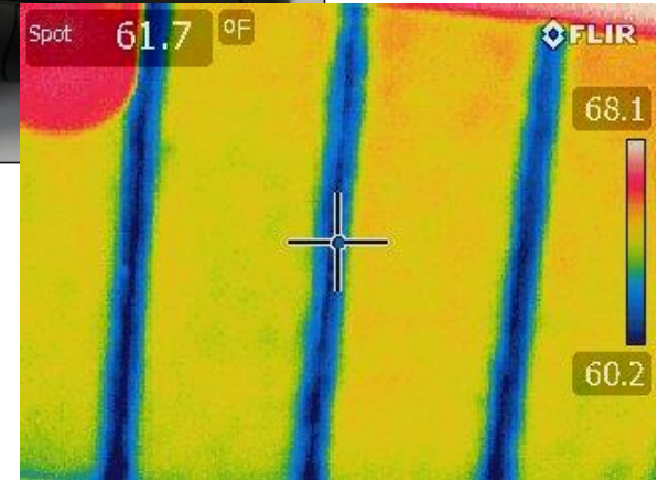
Right: Infrared Camera Photo (Underside of roof)
